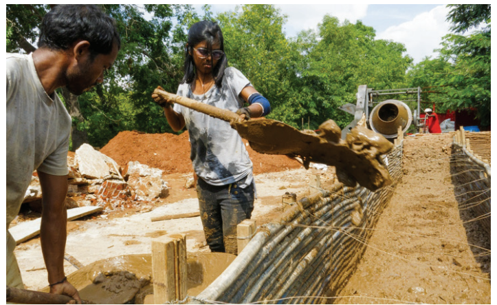
Constructing cob walls
