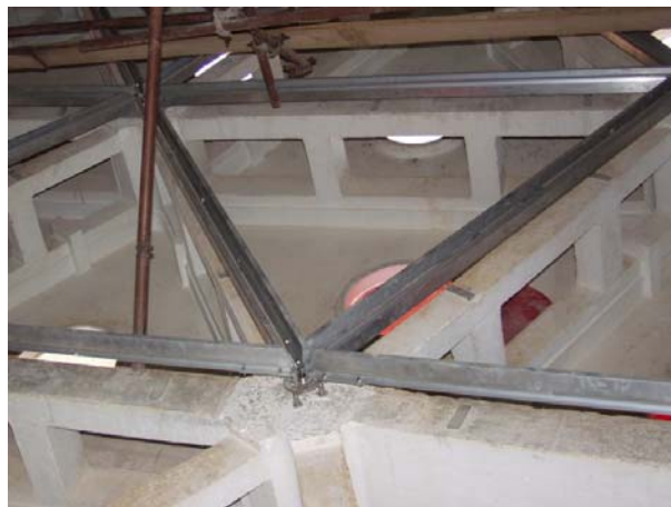
Frames which hold inner skin triangles
