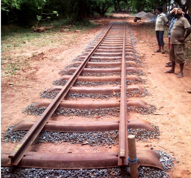
Prototype track laid in Auroville
