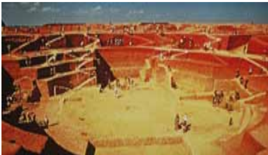
Excavation of the foundations for Matrimandir
