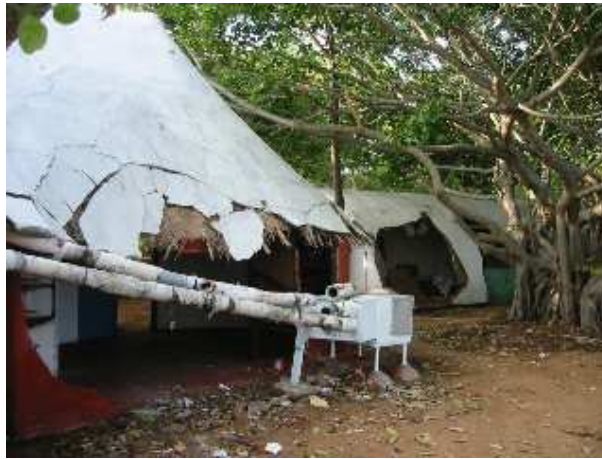
A shattered Auroville house in Sri Ma
